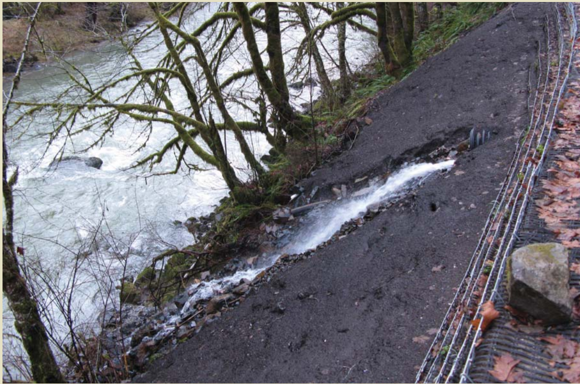
Figure 17. Compost over riprap at culvert after planting
