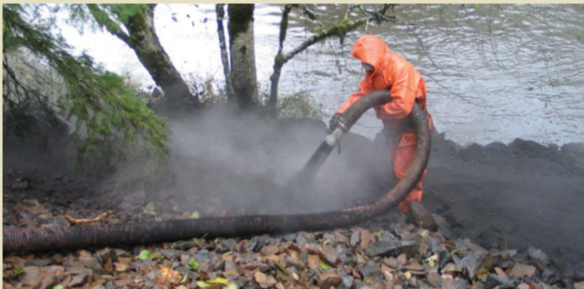
Figure 15. Application of compost over rip rap
