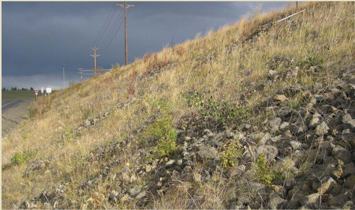
Figure 26. Setters Road rock mulch and revegetation
