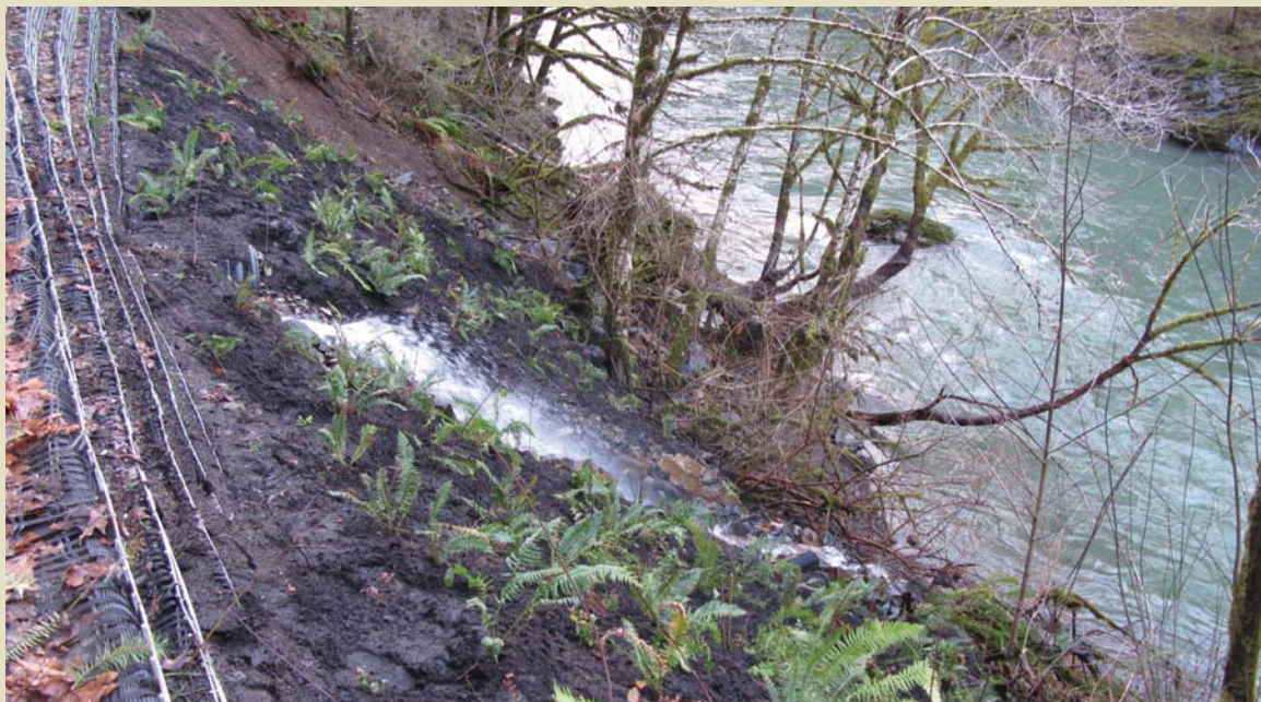
Figure 17. Compost over riprap at culvert after planting
