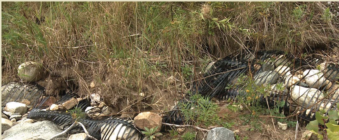
Figure 5. Geogrid sub-base stabilization planting near Wilmington, VT
