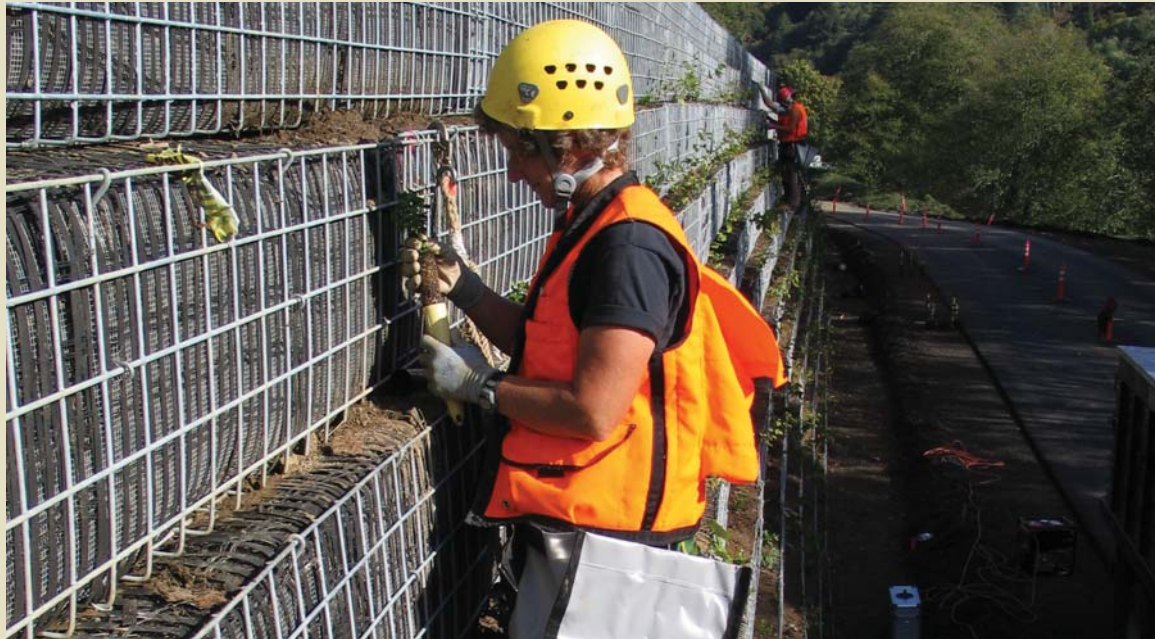
Figure 19. Plant installation on Mechanically Stabilized Earth Wall
