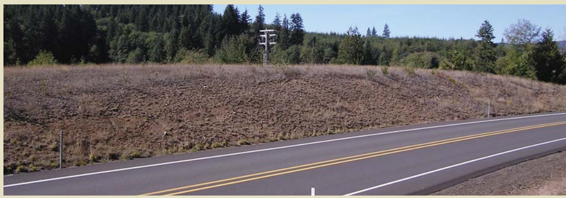
Figure 21. Example of hydroseeding without using blown in place mulch on Sandlake Road
