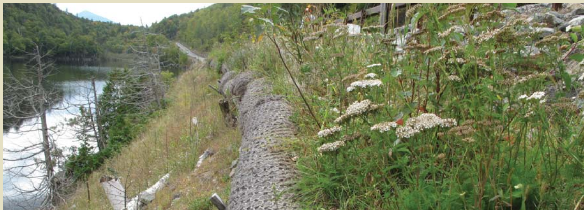
Figure 10. Coir log planting along Route 73 with Cascade Lakes in the background
