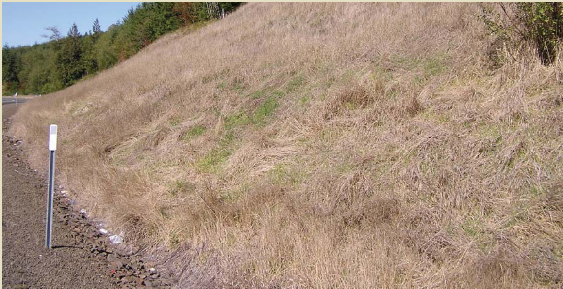
Figure 22. Example of seeding on steep slope and using blow-in-place compost on Sandlake Road
