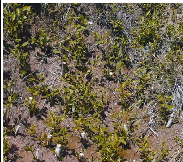
Figure 10.3.3.5. Hand-sticking cuttings at high densities is an option for saturated soils where the soils are too wet for installation of fascines or brushlayers.
