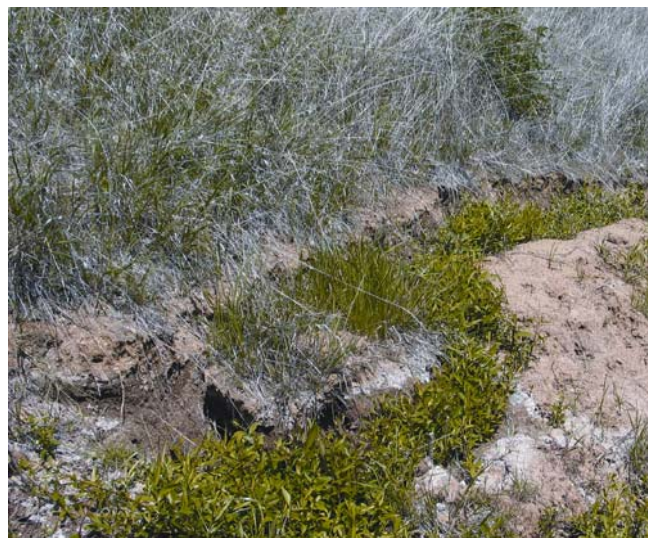
Figure 10.3.3.8. Slumps can be dewatered using live pole drains. Fascines were installed in the cracks of an active slump, directing the water downslope (lower left corner) and away from the slide to a more stable portion of the slope.
