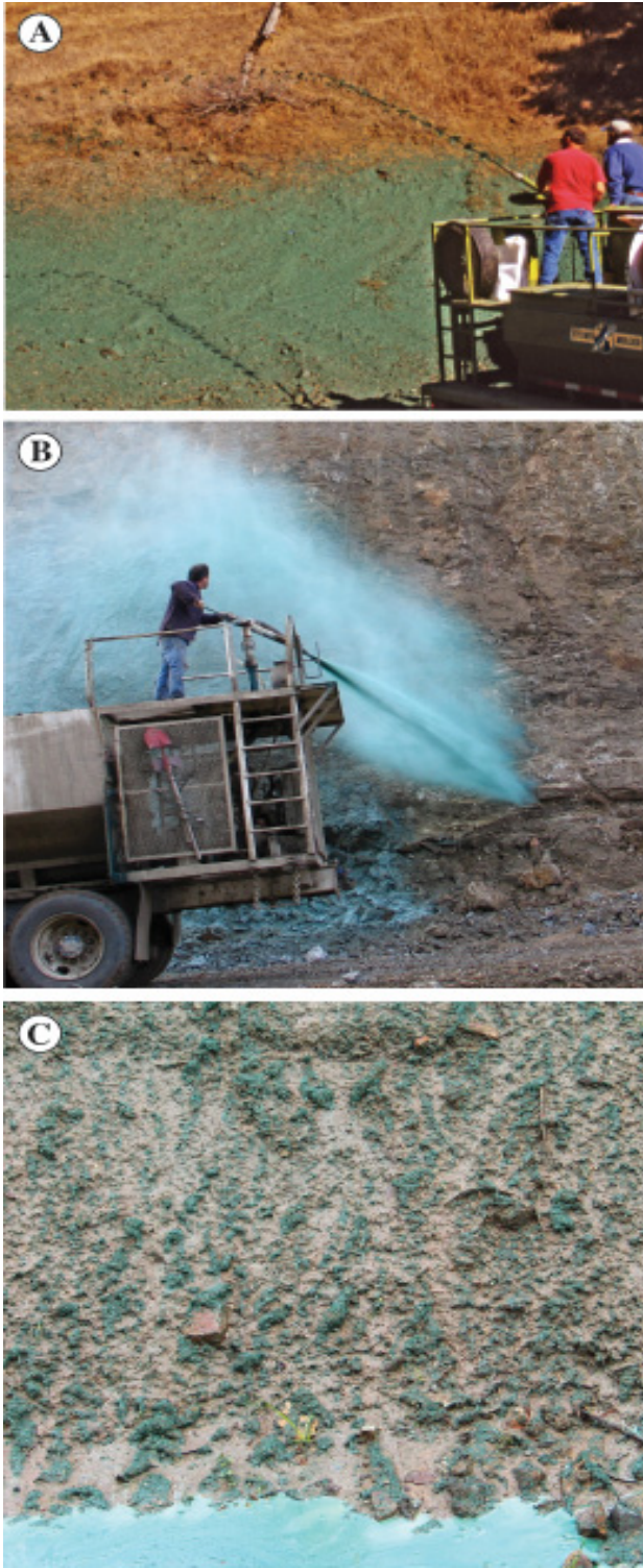
Figure 10.3.2.10. High viscosity tackifiers, mixed at manufacturer recommended rates, keep the slurry together during application using a “stream” nozzle (A). Low viscosity tackifiers, or slurries with low concentrations of tackifiers, do not hold together when applied and will drift with wind (B) or run off slopes (C).
