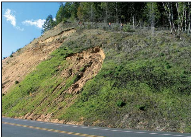
Figure 5.61 - This debris slide (noted by its shallow, steep appearance) took place two years after construction when the grass and forbs were fully established. Establishing shrub species, rather than grass and forb species, to steep, potentially unstable slopes would be better for long term stability because shrub species are deeper rooting and have higher root tensile strength.
