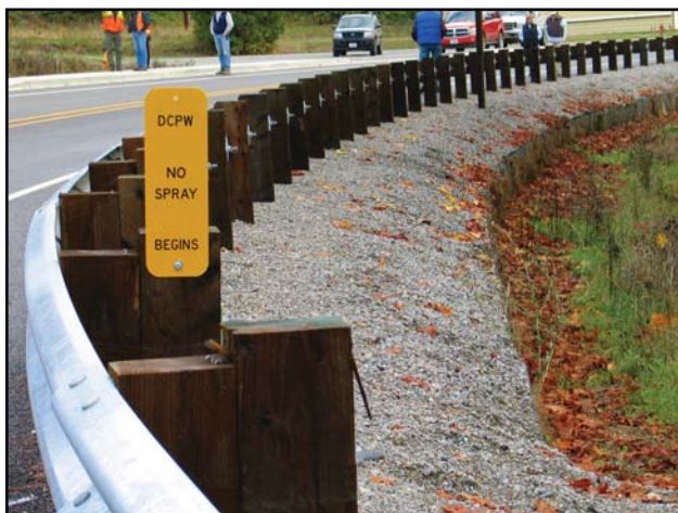
Figure 5.69 - Placing no-spray signs is a method of identifying areas to protect from herbicide application.
